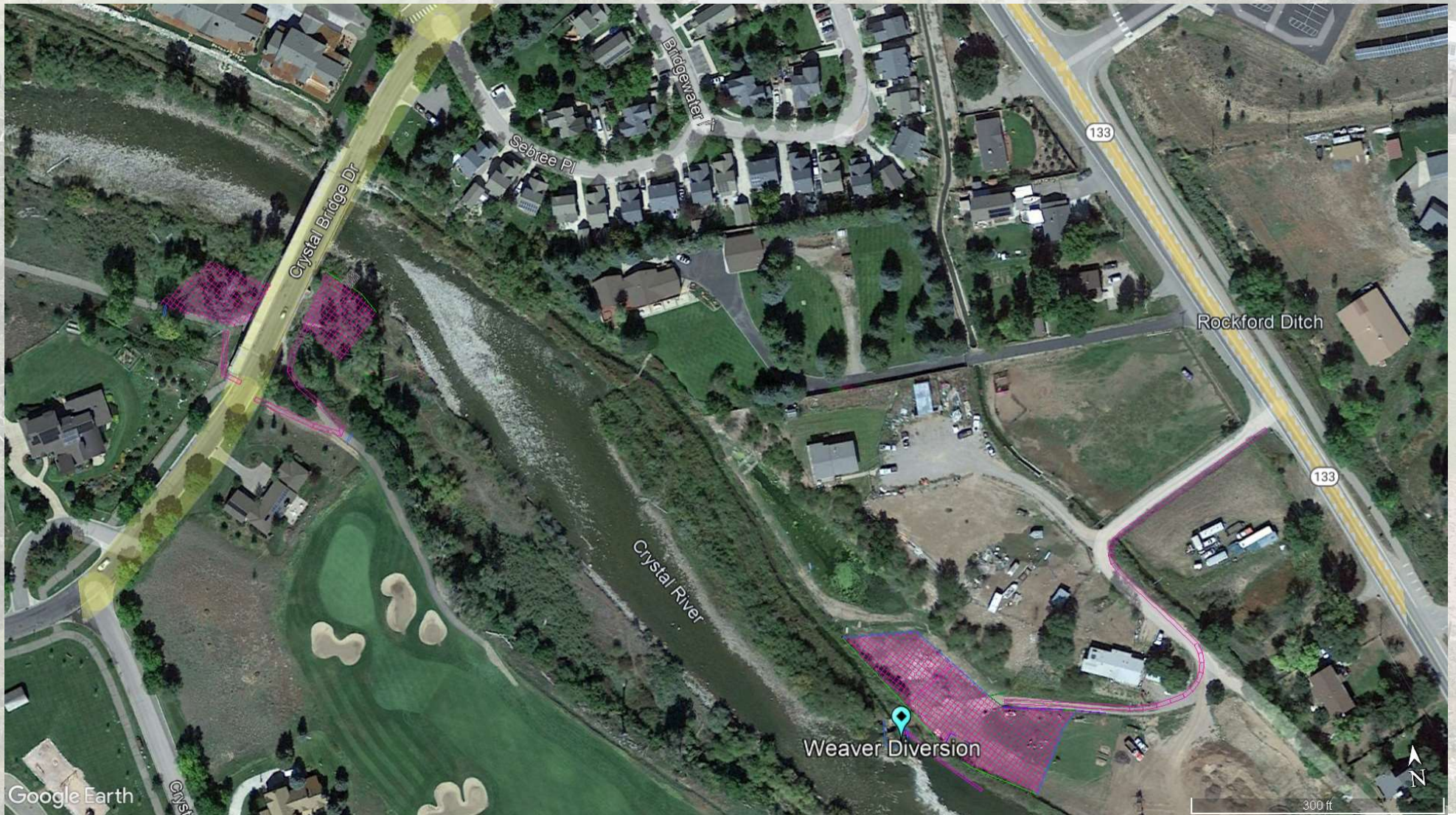
Crystal River Restoration Project
