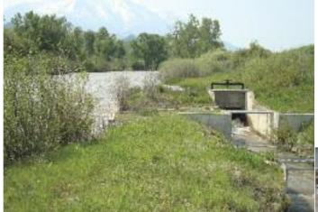
THE HEAD GATE AT THE CRYSTAL RIVER A mile up river, irrigation water leaves the Crystal and travels to RVR through the Bowles & Holland ditch. Each day during the season, a "ditch rider" inspects this weir and insures that the water flows unimpeded. The ditch rider also inspects for beaver activity and other environmental conditions which may negatively impact ditch operations. This weir also measures how much water RVR is drawing from the Crystal River.
