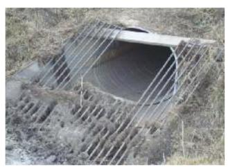
CULVERT WITH GRATE 8,000 lineal feet of our five ditches travel underground through culverts. Each culvert requires maintenance to insure that the irrigation water flows freely. The grates don't clean themselves after storms and mowing!
